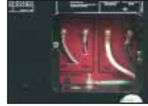
Large Input Reconnect Panel 208-575 Volts
