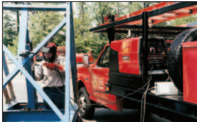
Make the Ranger 305G your portable welding station - General stick and downhill pipe, Touch-Start™ TIG, MIG, Flux-cored and AC generator to power lights, grinders or other power tools.
