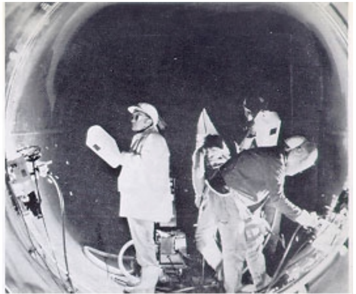
Weld position, vertical up.
