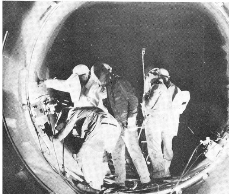
Automatic innershield welding with DCD ROL-O and Speed Weaver of a Penstock - 6 to 12 o'clock position, vertical up, overhead.
